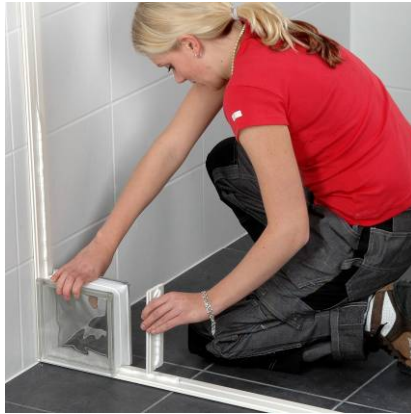
Glue the 18cm strips onto sides of the preceding blocks.
