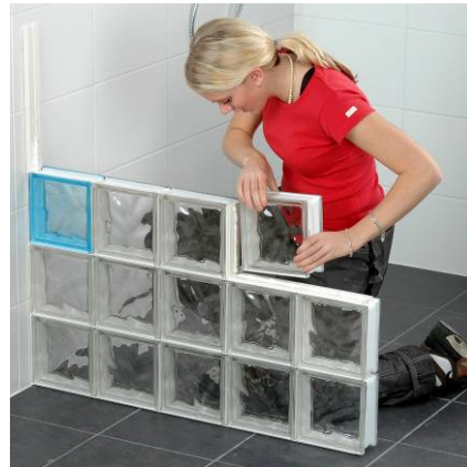
Glue the appropriate length of longer strips on to each horizontal course.
